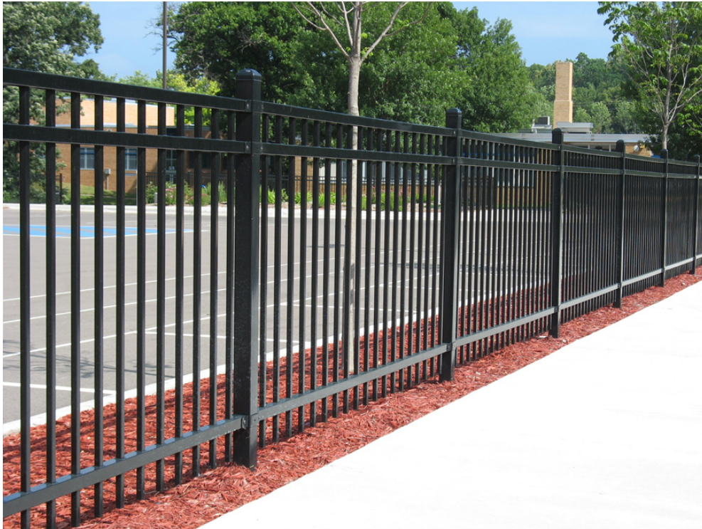
Figure 1- Decorative Steel Fence
