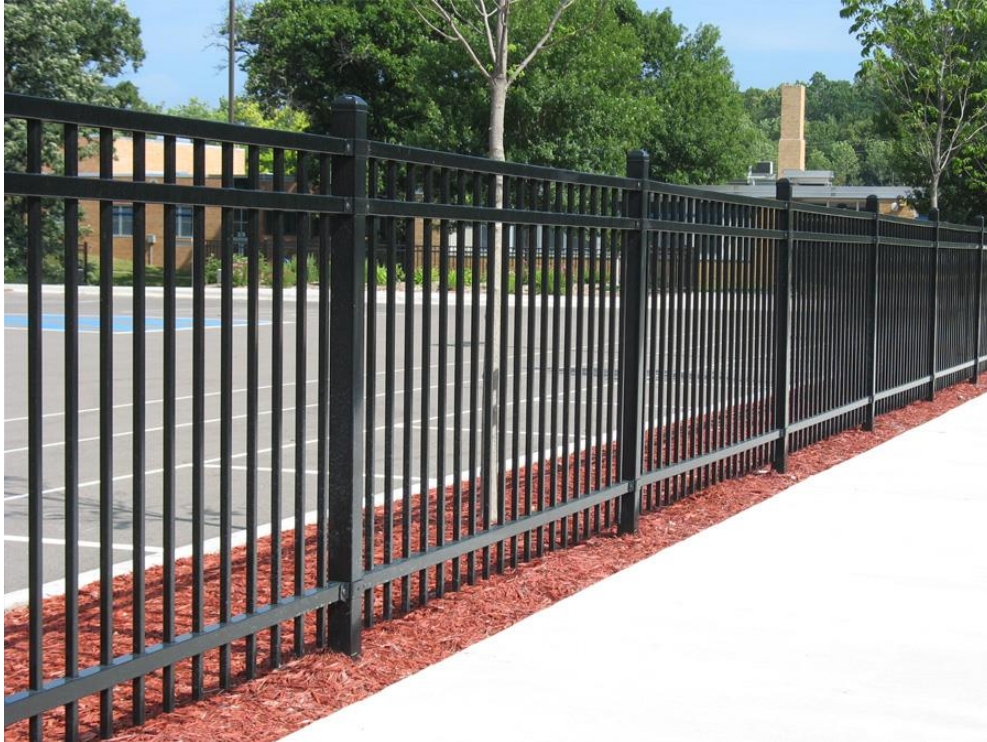
Figure 1- Decorative Steel Fence
