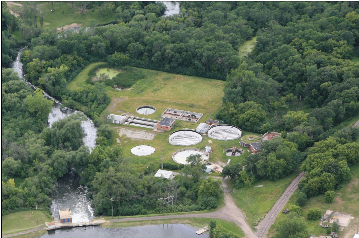
Old Waste Water Treatment Plant, Aerial Dated: Oct. 2009
