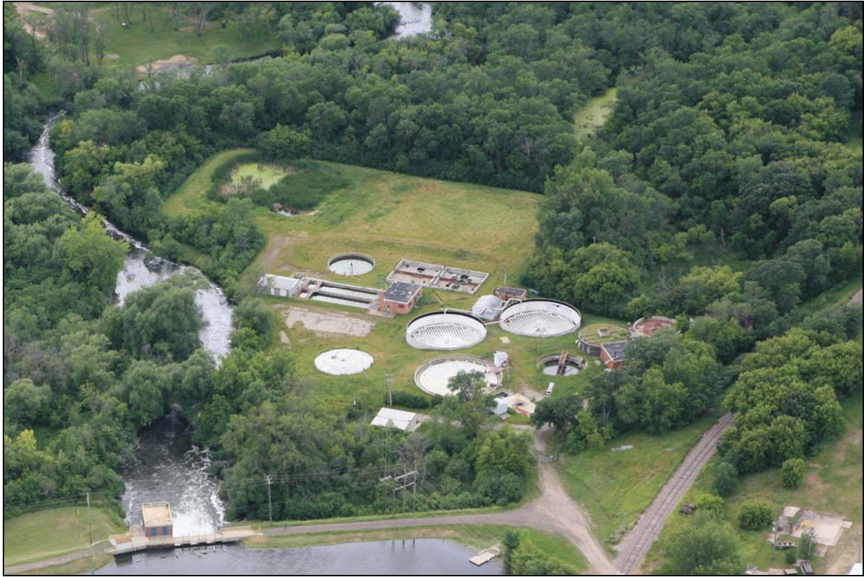
0.50 MGD Old Waste Water Treatment Plant, Aerial Dated: Oct. 2009
