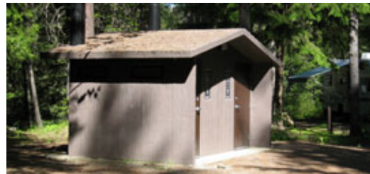
Prefabricated vault toilet structure common to campgrounds across the country.
