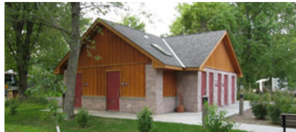
This MN DNR sanitation building is custom designed and provides toilets, showers, and a utility room.
