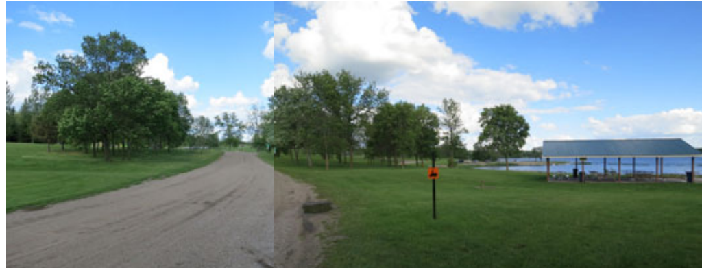
The existing entrance drive that provided access to the boat launch and picnic shelter will be removed.
