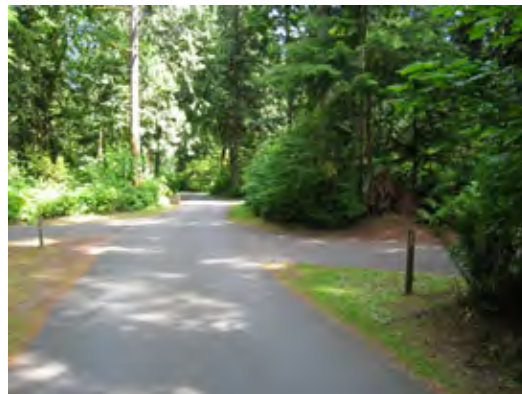
As this illustrates, at 12 foot 6 inches wide, the one-way roads through each of the camp loops will create an intimate feel yet be wide enough for even the largest rigs.
