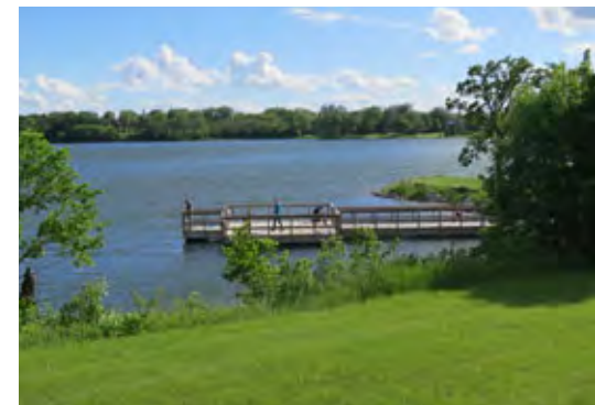
The existing fishing pier will be retained and is expected to remain a popular amenity.
