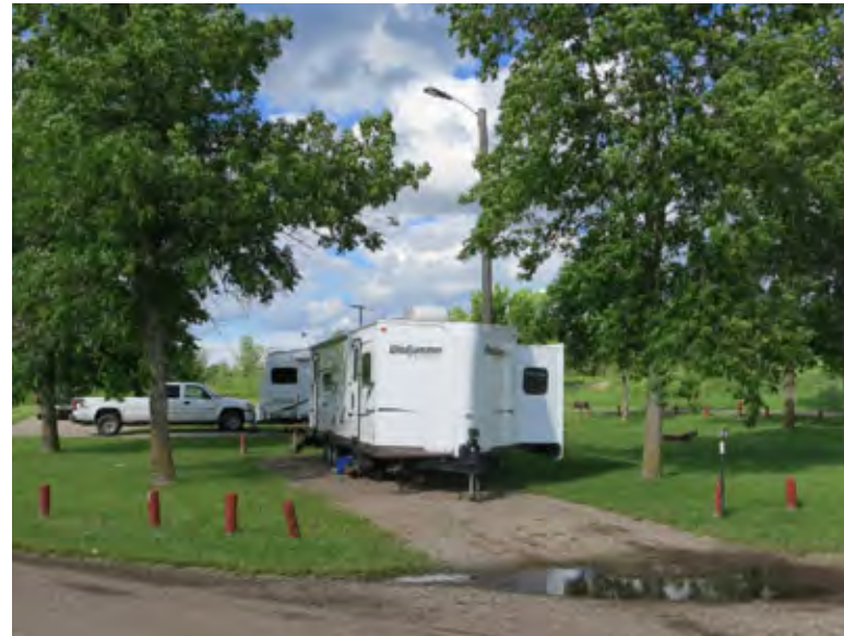
The existing campground is old and in need of upgrading.
