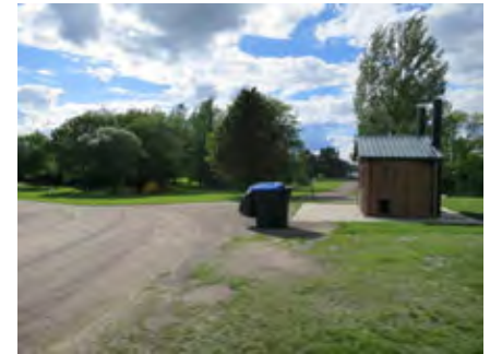
(N) The existing vault toilet is the only one available for campers.
