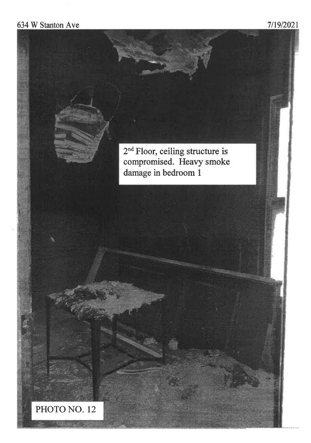
634 W Stanton Ave 7/19/2021 2<sup>nd</sup> Floor, ceiling structure is compromised. Heavy smoke damage in bedroom 2
