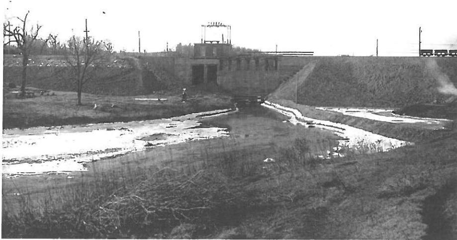
Fig. 87. OT-BUS-003. Pisgah Dam, upstream side nearing completion; note construction rail cars on embankment; 1918 photo by W. T. Oxley (Otter Tail Power Company Collection) (facing SW)
