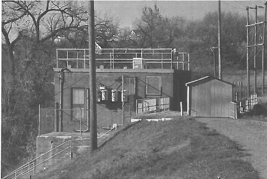
Fig. 94. OT-BUS-003. Pisgah Dam, southern elevation of powerhouse, embankment in foreground (facing NW)
