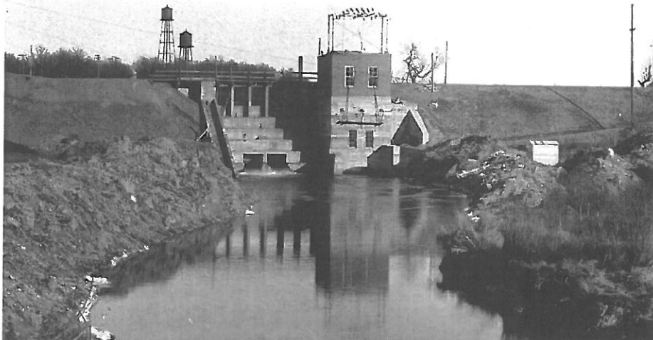
Fig. 86. OT-BUS-003. Pisgah Dam, downstream side nearing completion; 1918 photo by W. T. Oxley (Otter Tail Power Company Collection) (facing E)
