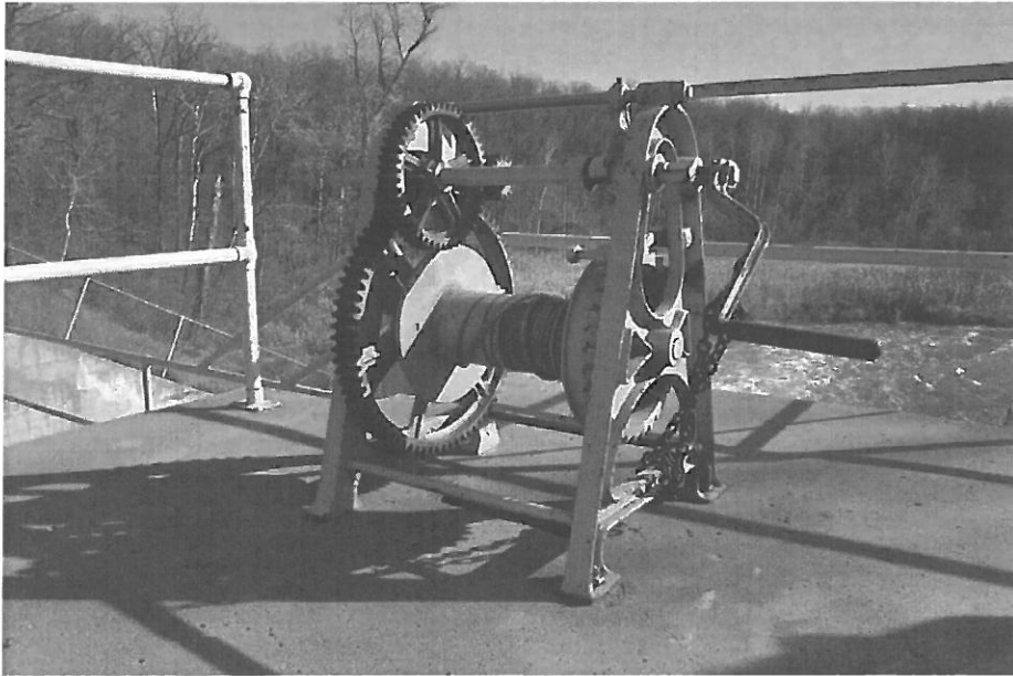
Fig. 118. OT-FRI-005. Taplin Gorge, Tainter gate mechanism on spillway (facing NE)
