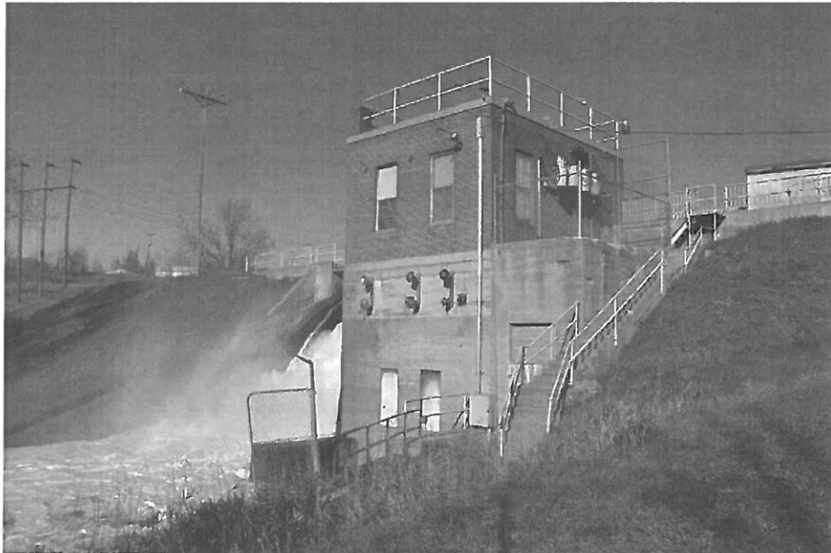
Fig. 96. OT-BUS-003. Pisgah Dam, dam and powerhouse (facing N)
