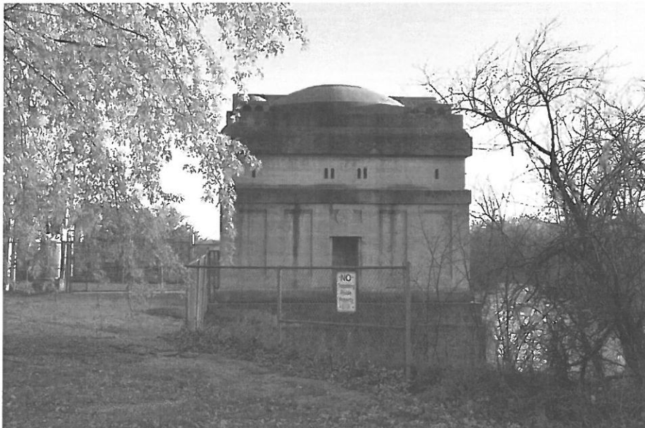
Fig. 131. OT-FRI-005. Taplin Gorge, northern elevation of powerhouse (facing S)
