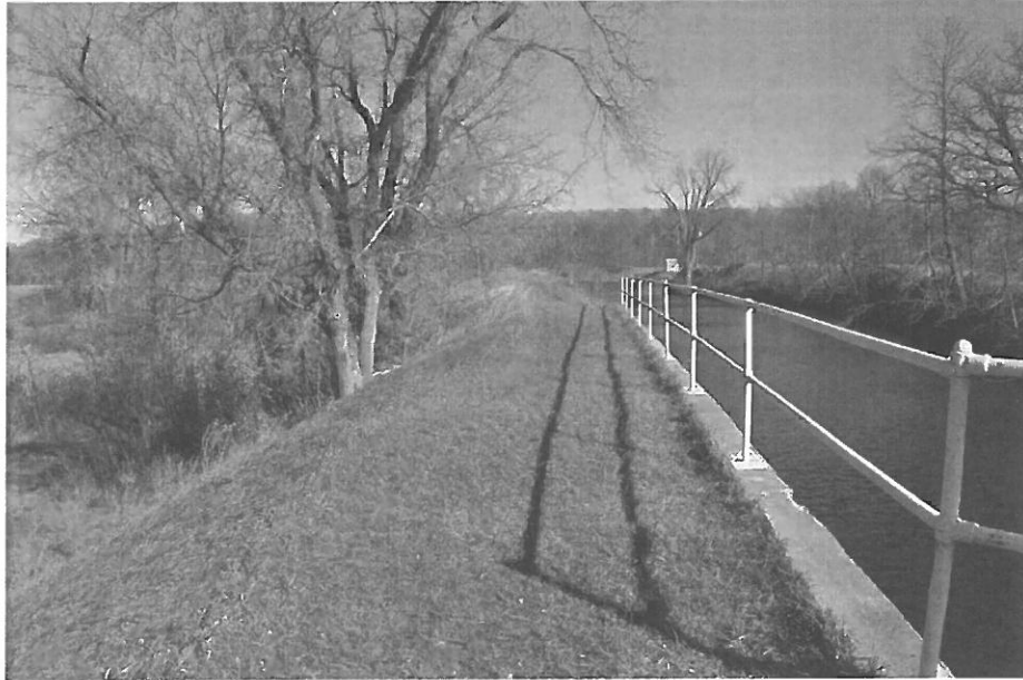
Fig. 122. OT-FRI-005. Taplin Gorge, northern side of diversion or power canal; manmade embankments form canal walls (facing E)
