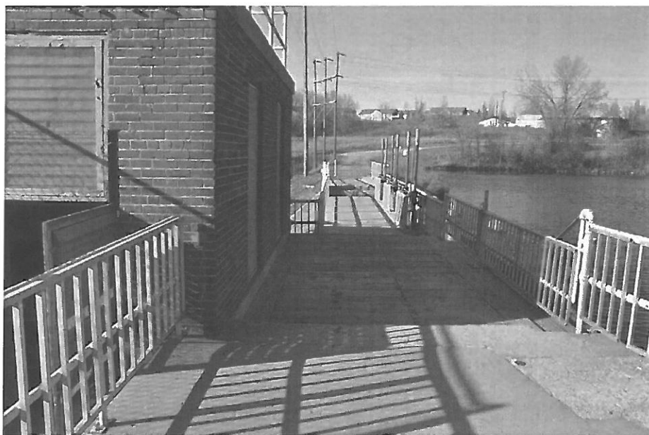
Fig. 99. OT-BUS-003. Pisgah Dam, powerhouse water intakes are immediately east of the powerhouse beneath the timber decking in the walkway (facing NW)
