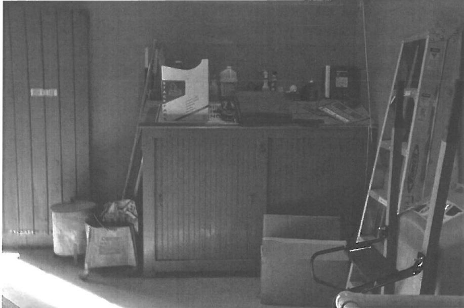
Fig. 135. OT-FRI-005. Taplin Gorge, powerhouse's wooden cupboard with slanted desk-like top for record-keeping (facing E)
