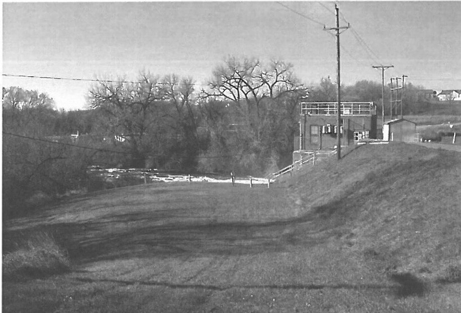
Fig. 93. OT-BUS-003. Pisgah Dam, dam and powerhouse from the south (facing NW)
