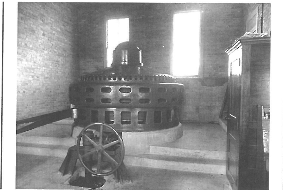
Fig. 89. OT-BUS-003. Pisgah Dam, powerhouse interior with Electric Machine Co. generator (still in place); 1921 photo by W. T. Oxley (Otter Tail Power Company Collection) (facing NE)
