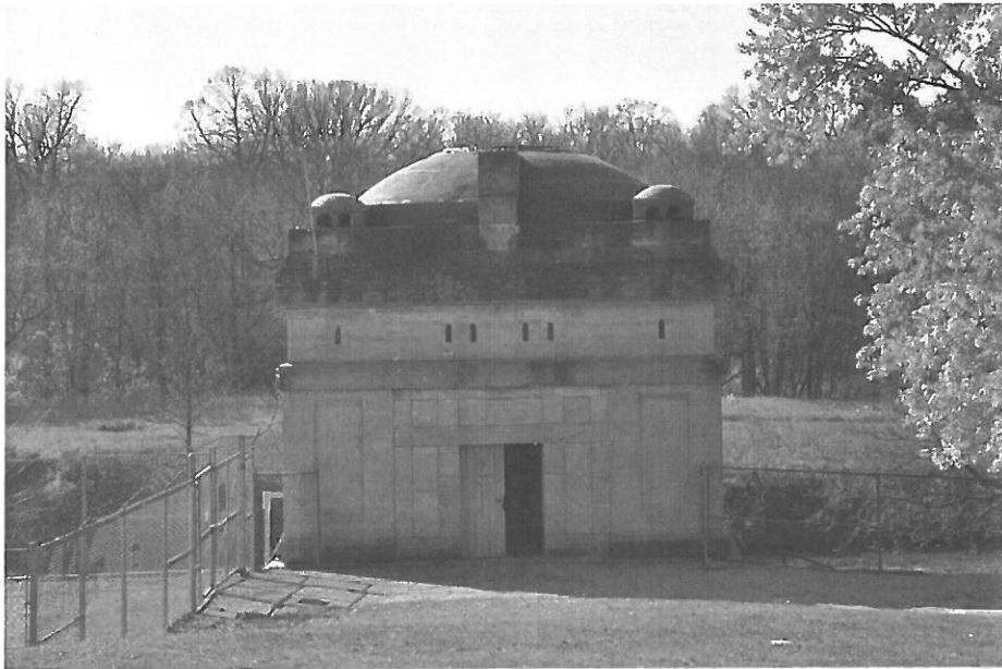
Fig. 128. OT-FRI-005. Taplin Gorge, eastern (main) facade of powerhouse; penstock is buried in the foreground (facing W)
