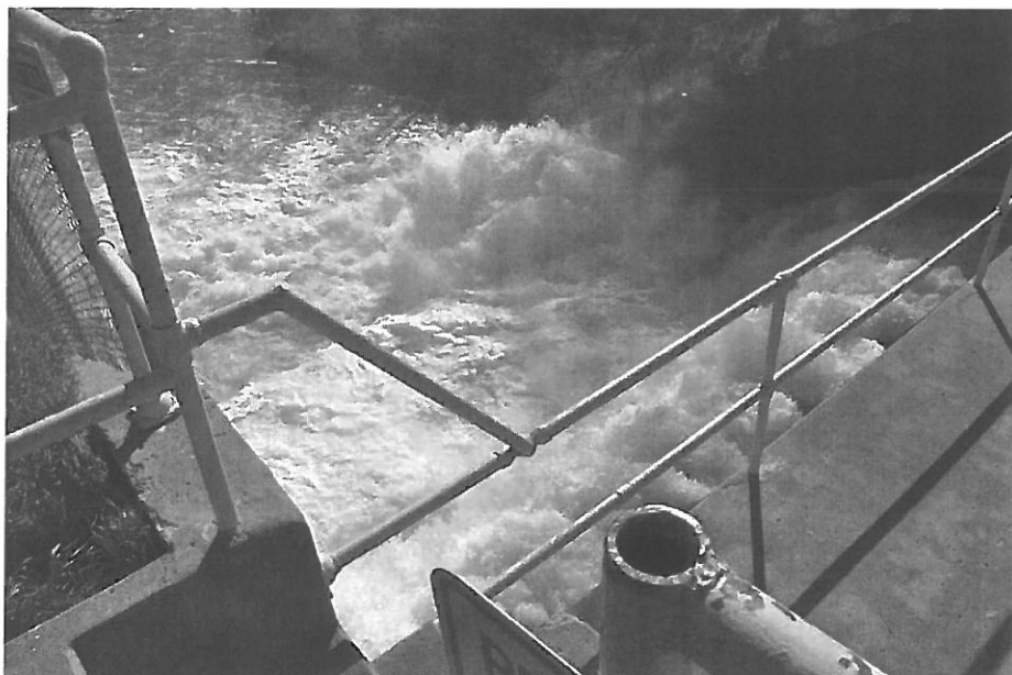
Fig. 116. OT-FRI-005. Taplin Gorge, dam spillway from the top (facing SW)
